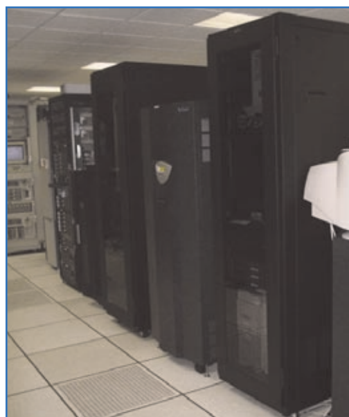
Existing Data Center
